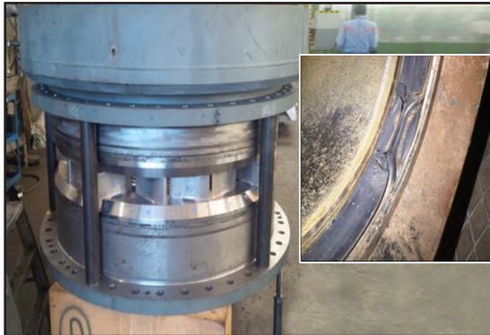
Wicket gate cylinder being rebuilt. Insert: damaged rubber u-cup seal
